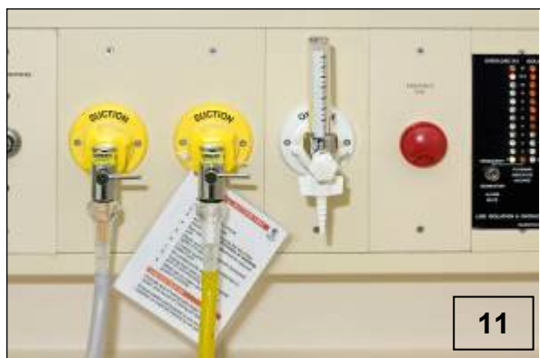
Figure 11: High flow suction regulator setup secondary to emergency suction.
