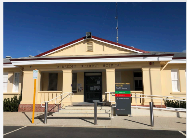
Merredin District Hospital
